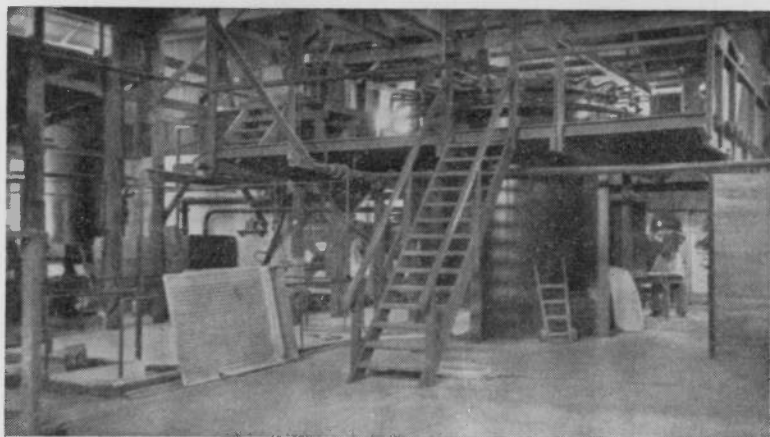
Fig. 1. Merrill-Crowe Precipitation Plant.
