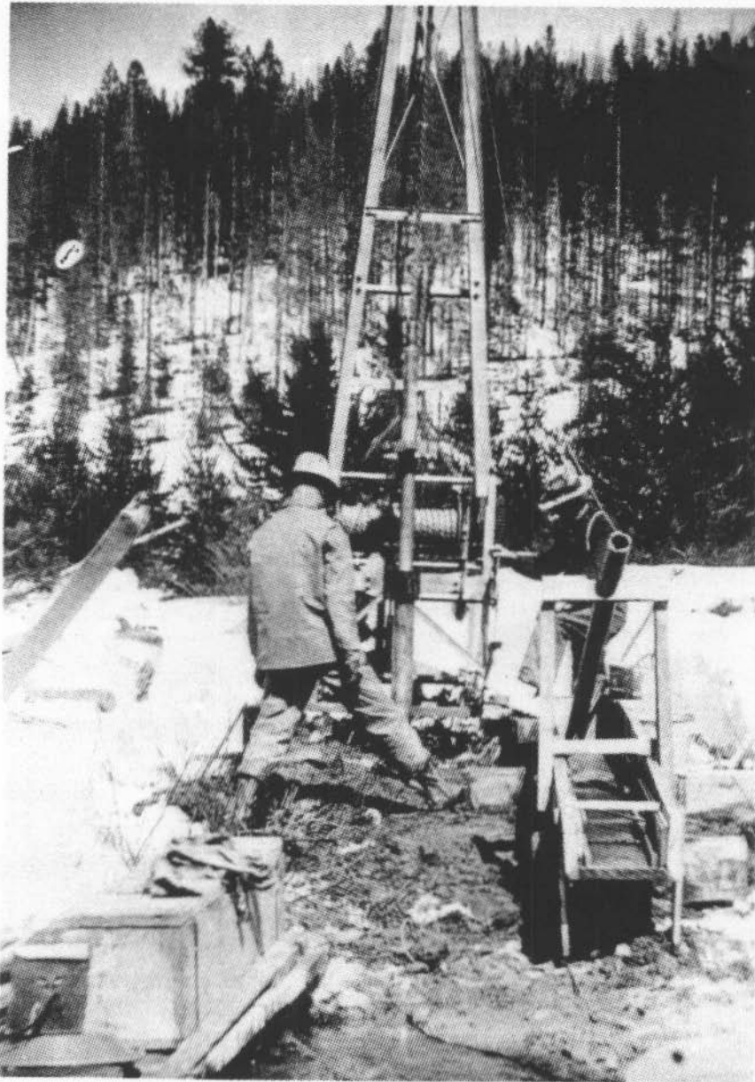
FIGURE 9. — Hillman 4-inch Airplane drill. This compact, skid-mounted machine is widely used for reconnaissance-type prospecting.
