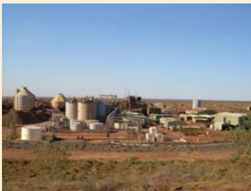
Granites processing facility
