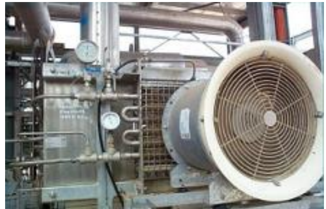
Figure 1. Forced Convection Air Fin Cooler
