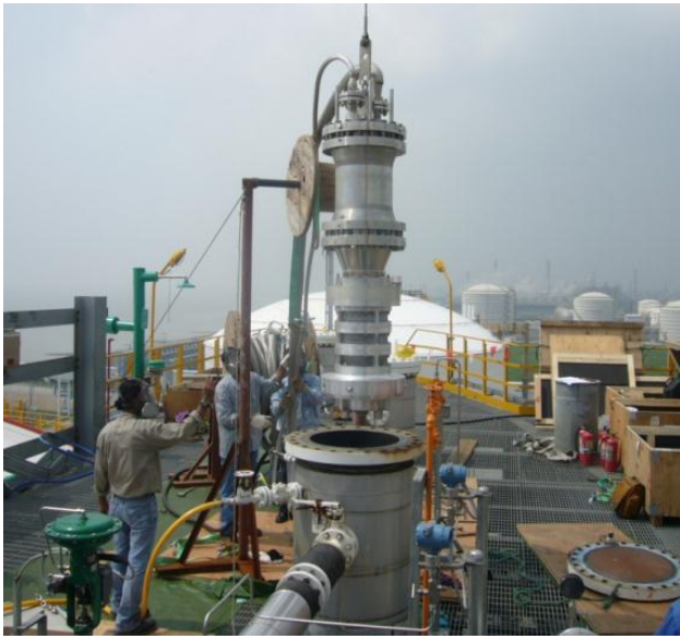
Figure 1: Installation of a Removable Type Ammonia Pump with Magnetic Coupling
