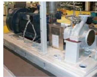
Figure 3: Flat deck type with a mounted sloped gutter drain
