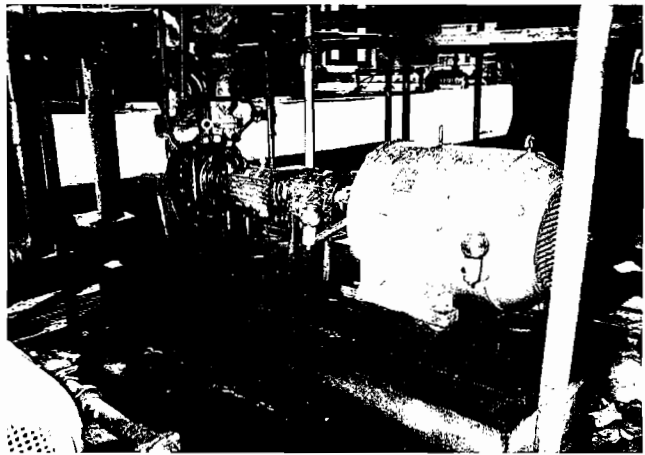
Figure 5. Simple Baseplate Design with Sloping Flat Center Drain. This design avoids the trash-collecting tendencies of that shown in Figure 4.
