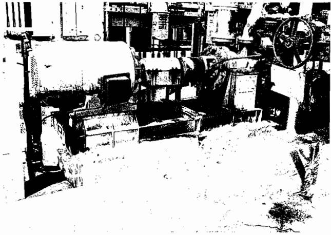
Figure 4. Open-Top Frame Design for Pump Baseplate. This design promotes trash accumulation, and should be avoided.
