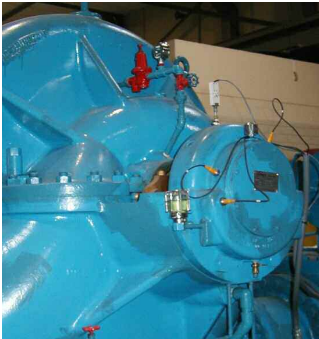
Figure 2. Pump Bearing Housing with Mounted Accelerometers.
