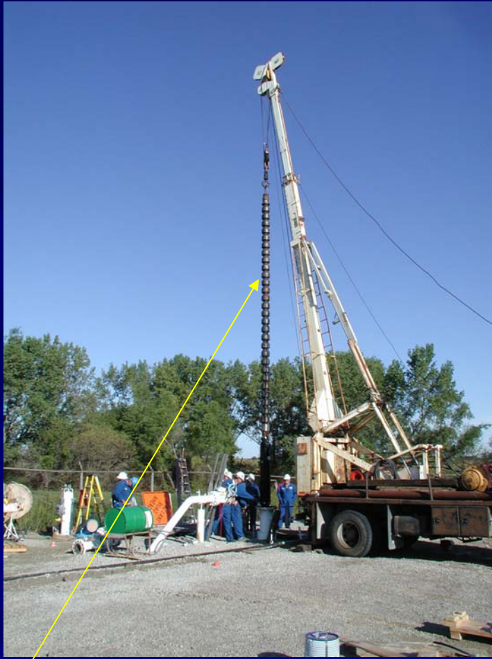
Pump being installed into caisson
