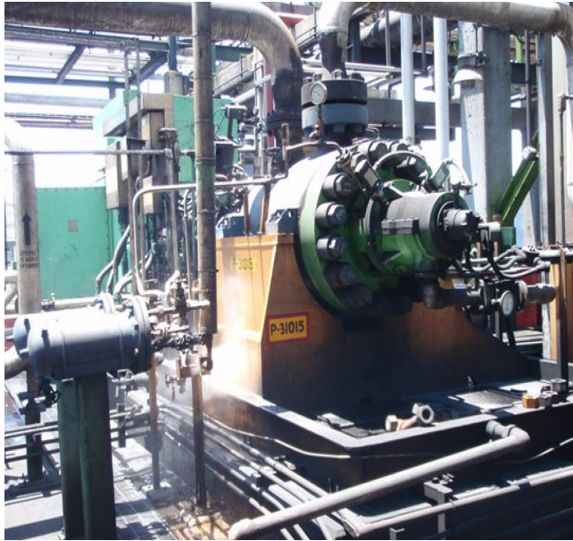
Figure 7. Water Jet Pump Train with Variable Speed Geared Coupling.
