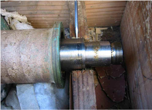
Figure 3. Fretting Damage on Shaft from Lip Seal.
