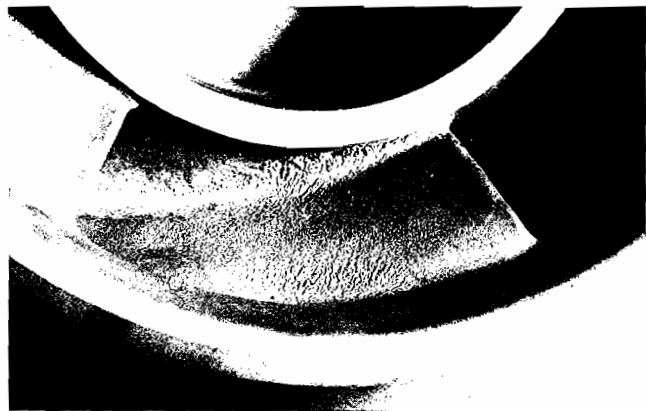
Figure 2. Cavitation Damage on 12 × 18 CA Suction Impeller. The damage accumulated on this impeller occurred over a period of about 18 months operation. It is considered at the end of its operational life. No pressure (or hidden side) damage was observed.
