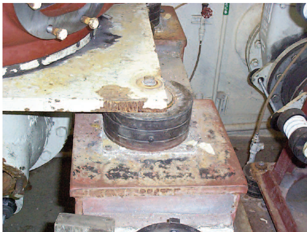
Figure 8. Original Pneumatic Baseplate Isolator.
