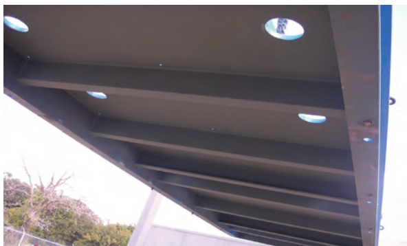
Figure 4. Under Side of Base Plate.
