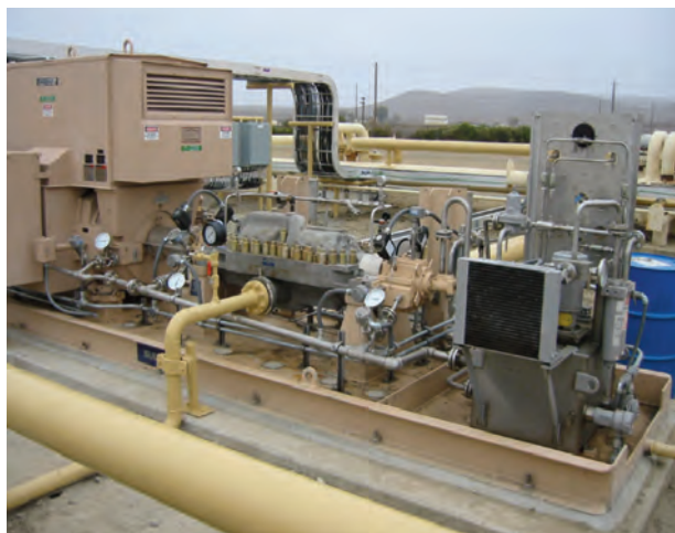
Figure 33. Pump Prepared for First Start.
