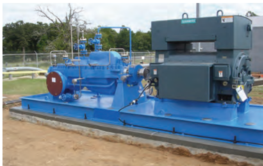
Figure 10. Base with Motor Mounted in the Field, not in the Factory.
