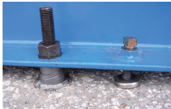
Figure 6. Anchor Bolts and Leveling Jackscrew.
