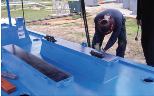
Figure 8. Base Plate Tightening after Base Level on Pads Achieved.
