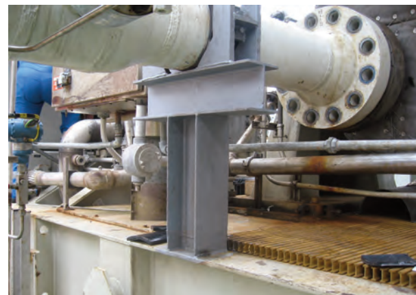
Figure 18. Check for Pipe Strain.
