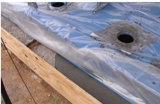
Figure 15. Initial Grout Pour.
