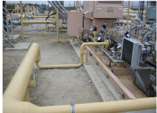
Figure 17. Main Piping.
