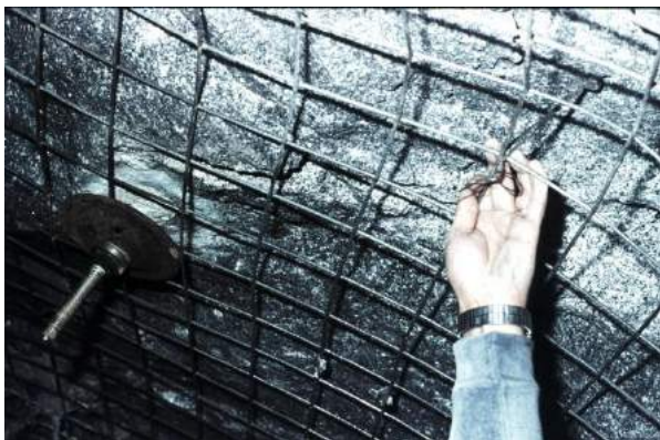
Figure 8: Welded wire mesh, firmly attached to the rock surface, provides excellent reinforcement for shotcrete.
