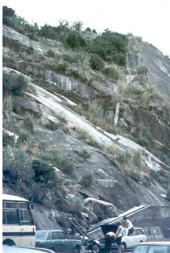
Figure 4: The failure surface defined by a sheet joint surface on which a small slide occurred during blasting of the original cut slope for the Sau Mau Ping Road. The potentially unstable slope under consideration is visible in the background.
