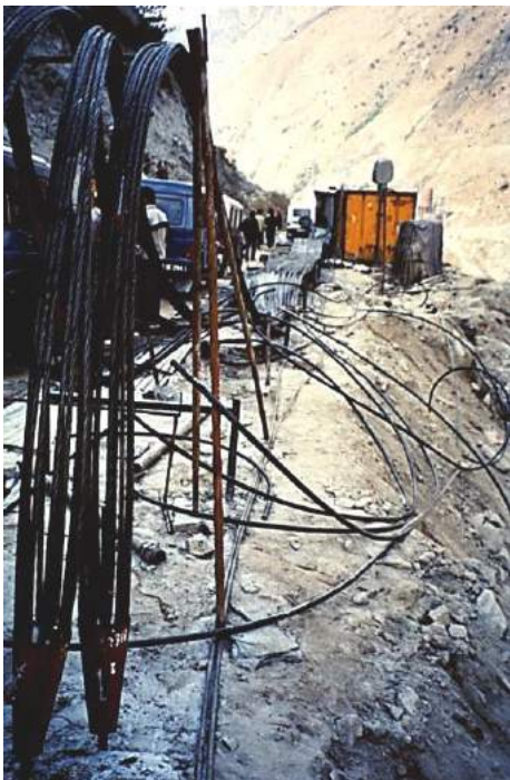
Figure 16: Drilling machine for the installation of 40 m long reinforcing cables in 150 mm diameter holes in a dam excavation.
