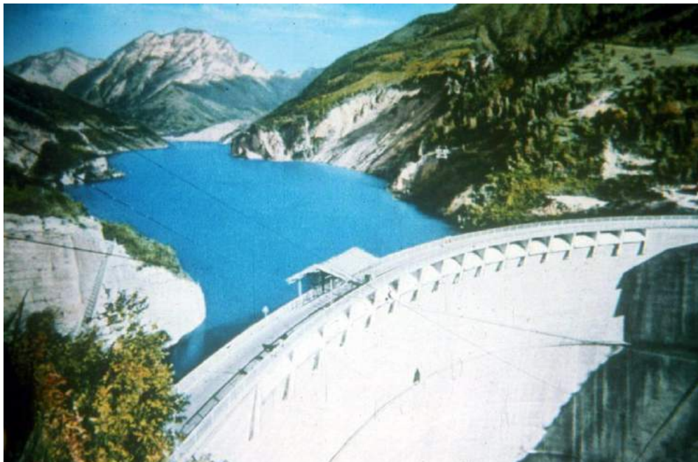
Figure 2a: The Vajont dam during impounding of the reservoir. In the middle distance, in the centre of the picture, is Mount Toc with the unstable slope visible as a white scar on the mountain side above the waterline.
