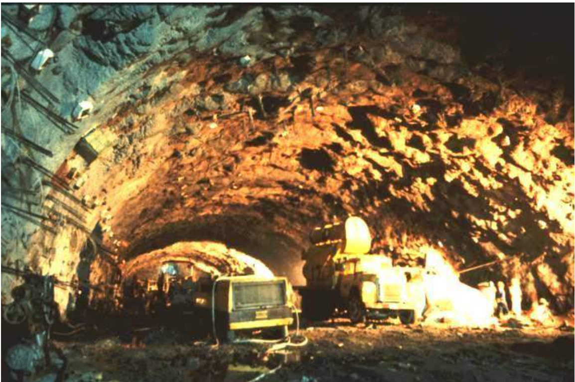
Figure 19: Completed excavation of the cavern arch.
