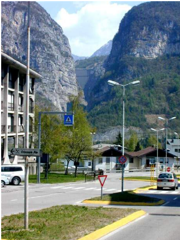
Figure 2e: The remains of the Vajont dam perched above the present town of Longarone. Photograph by Mark Diederichs, 2003.
