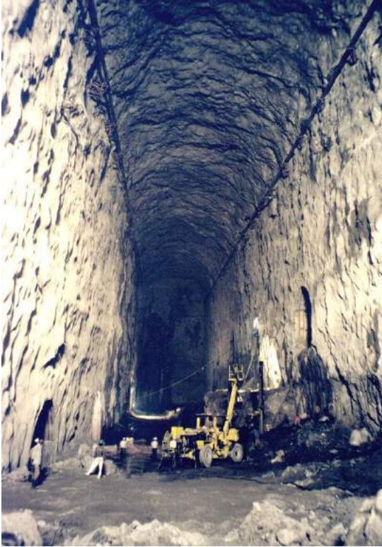
Figure 22: Partially completed 20 m span, 42.5 m high underground powerhouse cavern of the Nathpa Jhakri Hydroelectric Project in Himachel Pradesh, India. The cavern is approximately 300 m below the surface.
