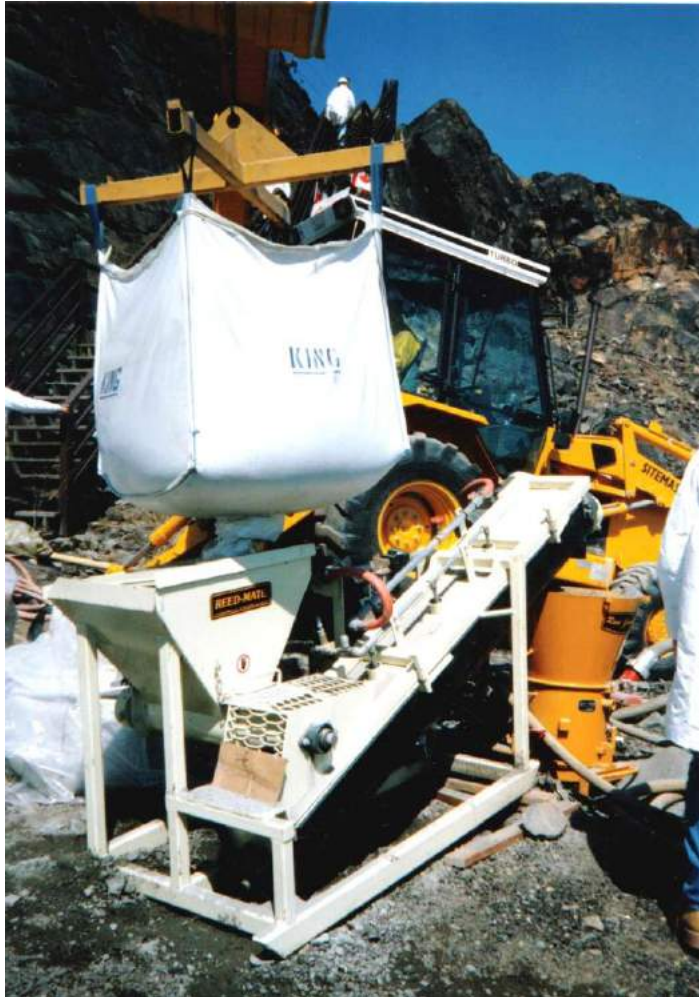
Figure 3: Bagged pre-mixed dry shotcrete components being delivered into a hopper feeding a screw conveyor, fitted with a pre-dampener, which discharges into the hopper of a shotcrete machine
