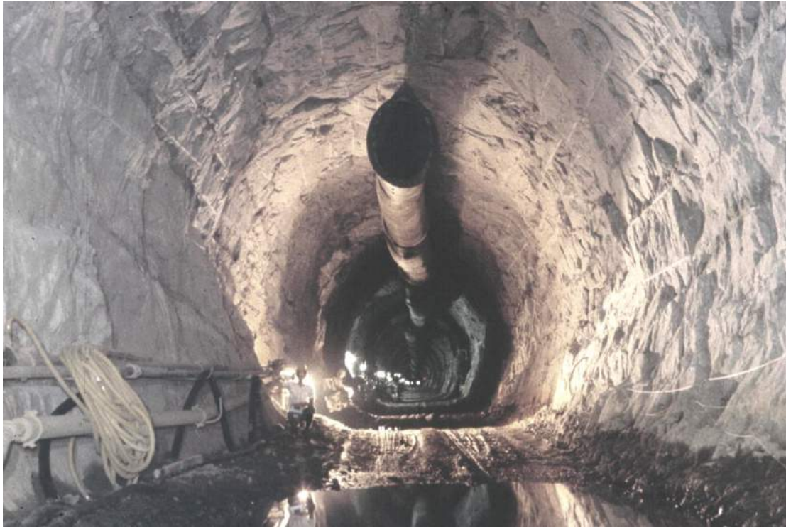
Figure 5: Results achieved using well designed and carefully controlled blasting in a 19 foot diameter tunnel in gneiss in the Victoria hydroelectric project in Sri Lanka. Note that no support is required in this tunnel as a result of the minimal damage inflicted on the rock. Photograph reproduced with permission from the British Overseas Development Administration and from Balfour Beatty - Nuttall.
