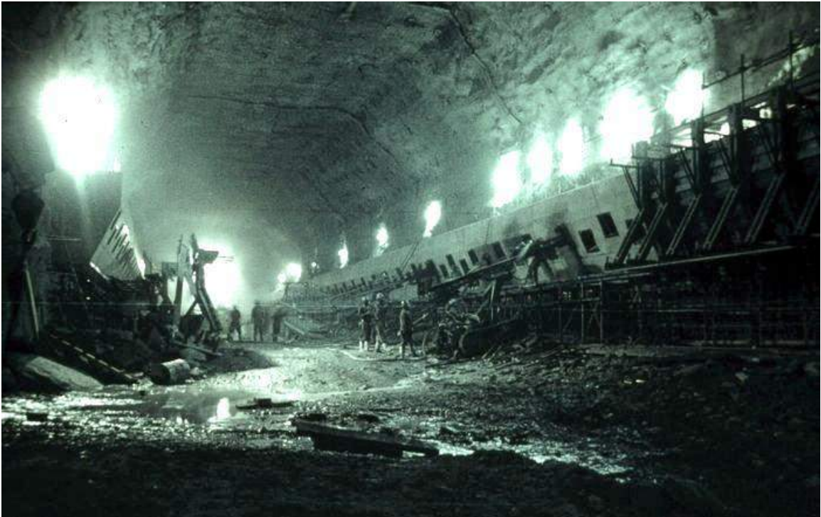
Figure 26: Cast in place concrete crane beam being anchored to the sidewall of the power cavern of the Drakensberg Pumped Storage Project in South Africa.
