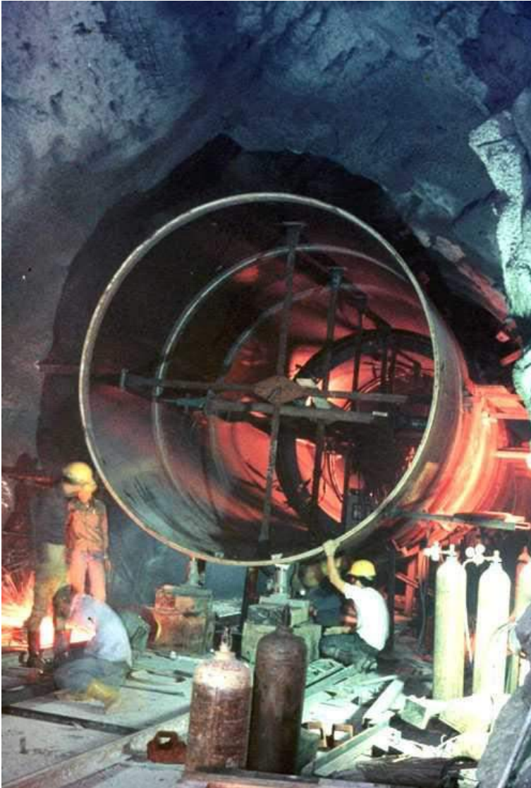
Figure 13: Installation of steel lining in a pressure tunnel in a hydroelectric project.
