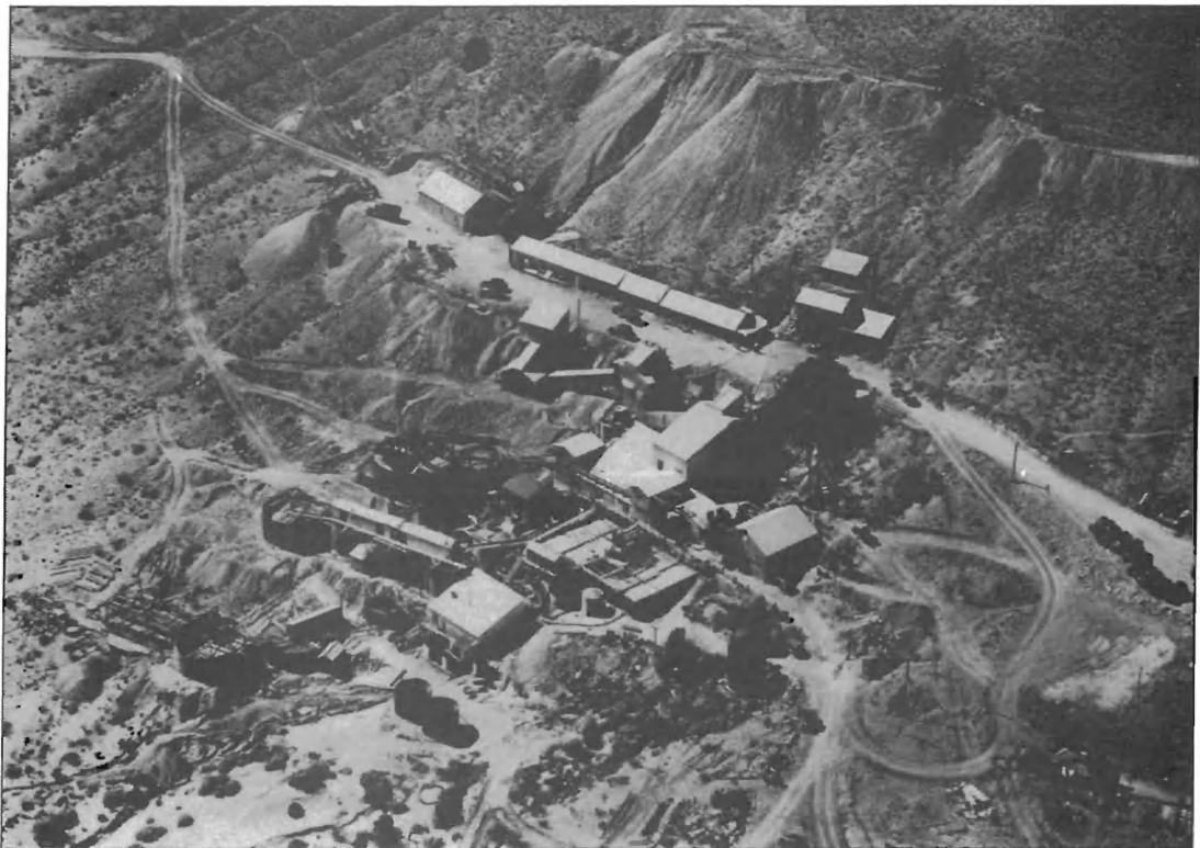
FIGURE 13.- Tropic mine and mill.
