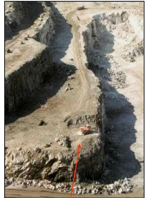
Prior bench level sub-drill zone removed
