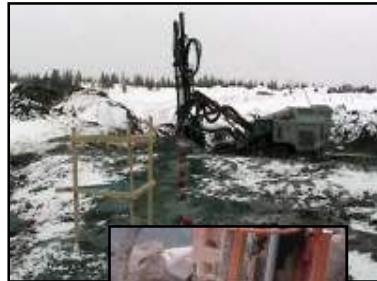
Drill-hole positioning, alignment and levelling
