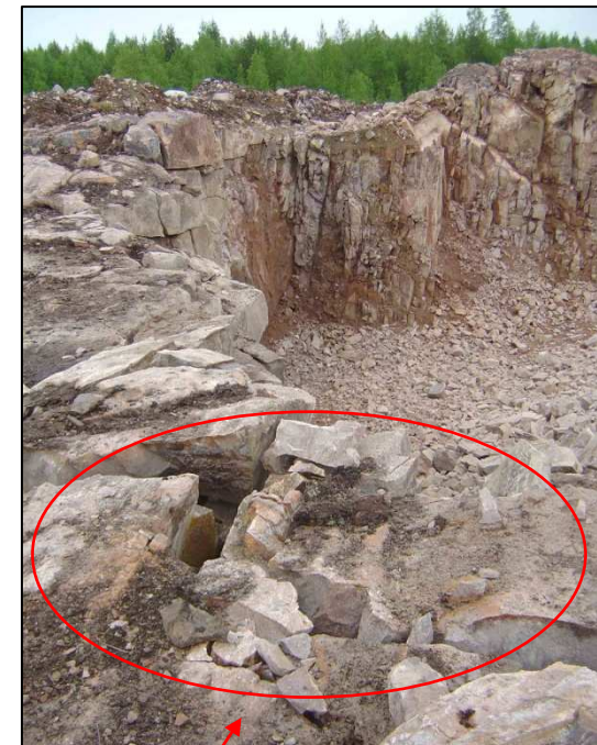
Side-break due to open corner damage
