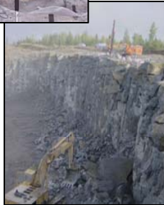
Re-drill crossed shotholes and clean toe area
